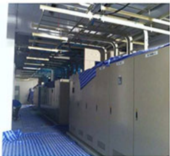
Inverter 2 kW and Soft start 250 kW Cabinet 4 X 3 kW
