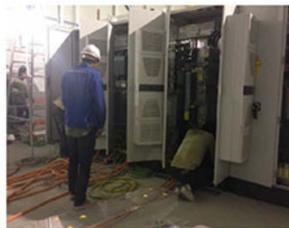
Inverter 2 kW and Soft start 250 kW Cabinet 4 X 3 kW
