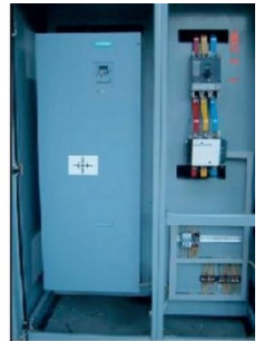
Inverter cabinet 4 X 3 kW
