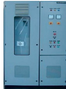
Inverter cabinet 4 X 3 kW
