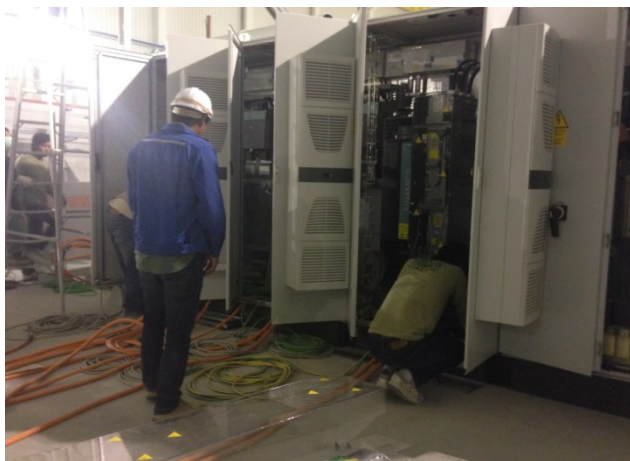
Inverter 2 kW and Soft start 250 kW Cabinet 4 X 3 kW
