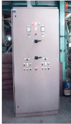
Inverter cabinet 4 X 3 kW
