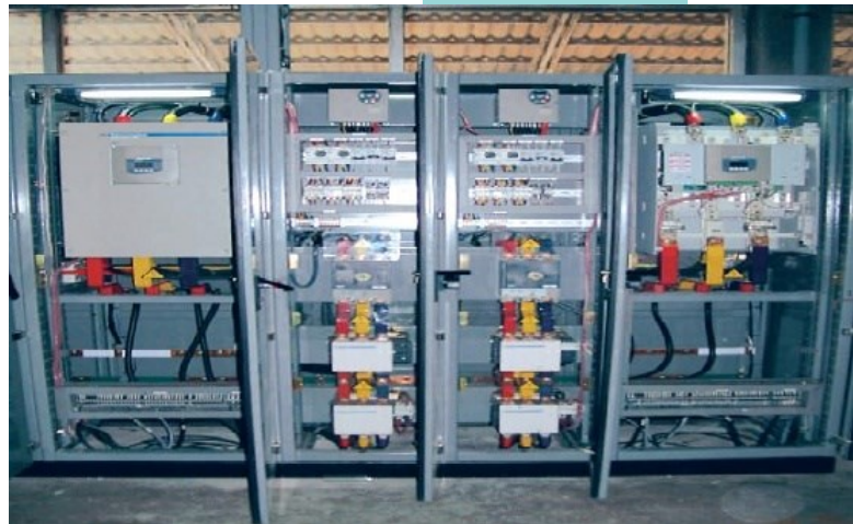
Inverter 2 kW and Soft start 250 kW Cabinet 4 X 3 kW
